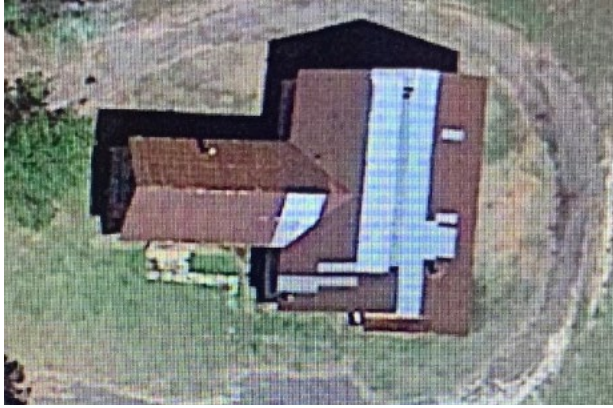
Current roof. Light color is modern metal replacement.
