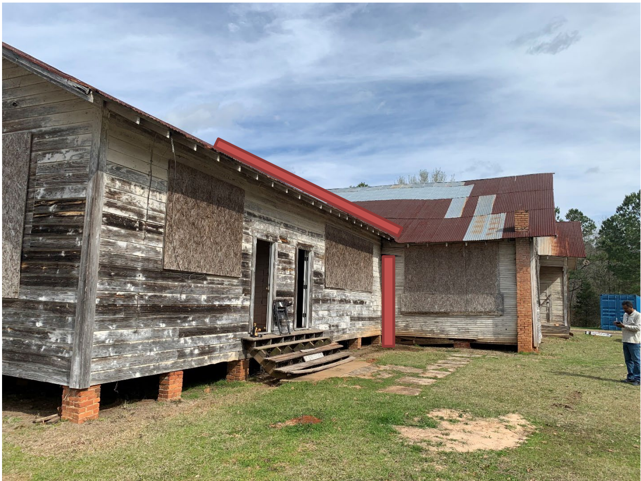
1930 West Wing Addition on left, 1925 Original Building on right.
