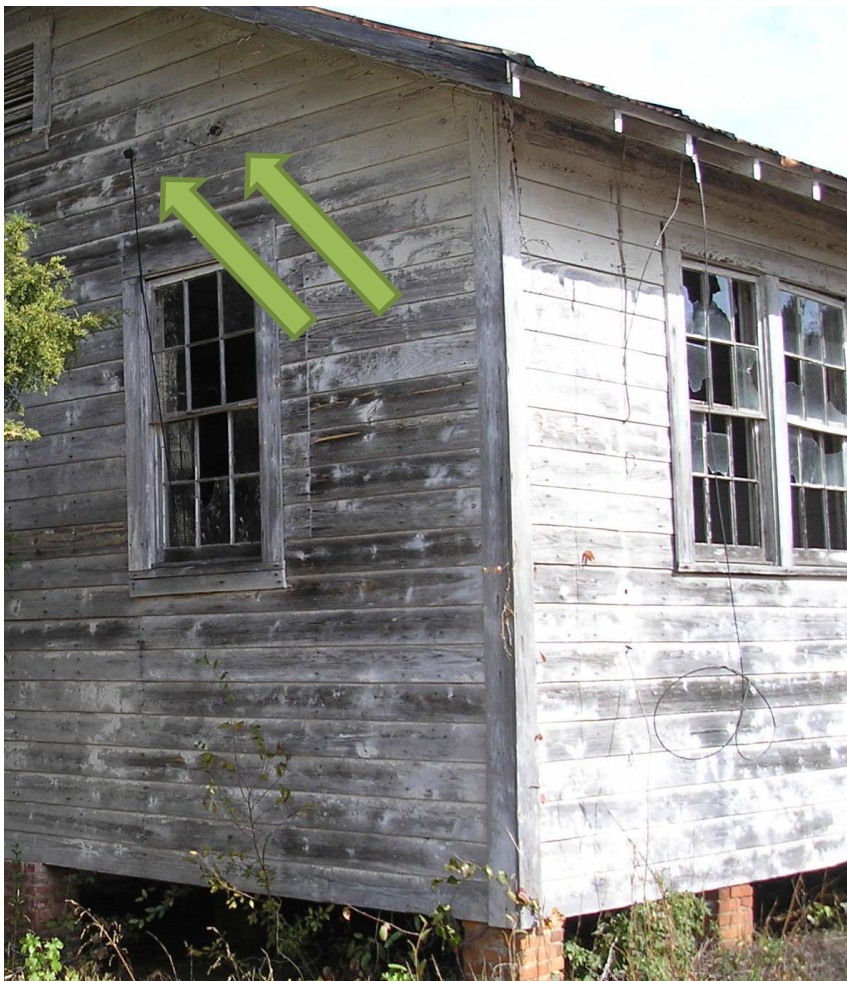
Probable 1930 service entry.
