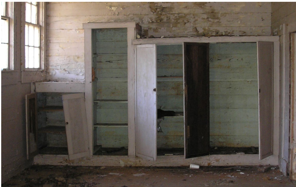
1925 Building. Room 104 – South end of room.
