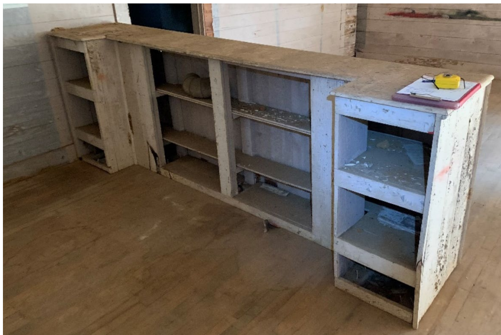
1930 West Wing, Room 111. 2023 photograph.
