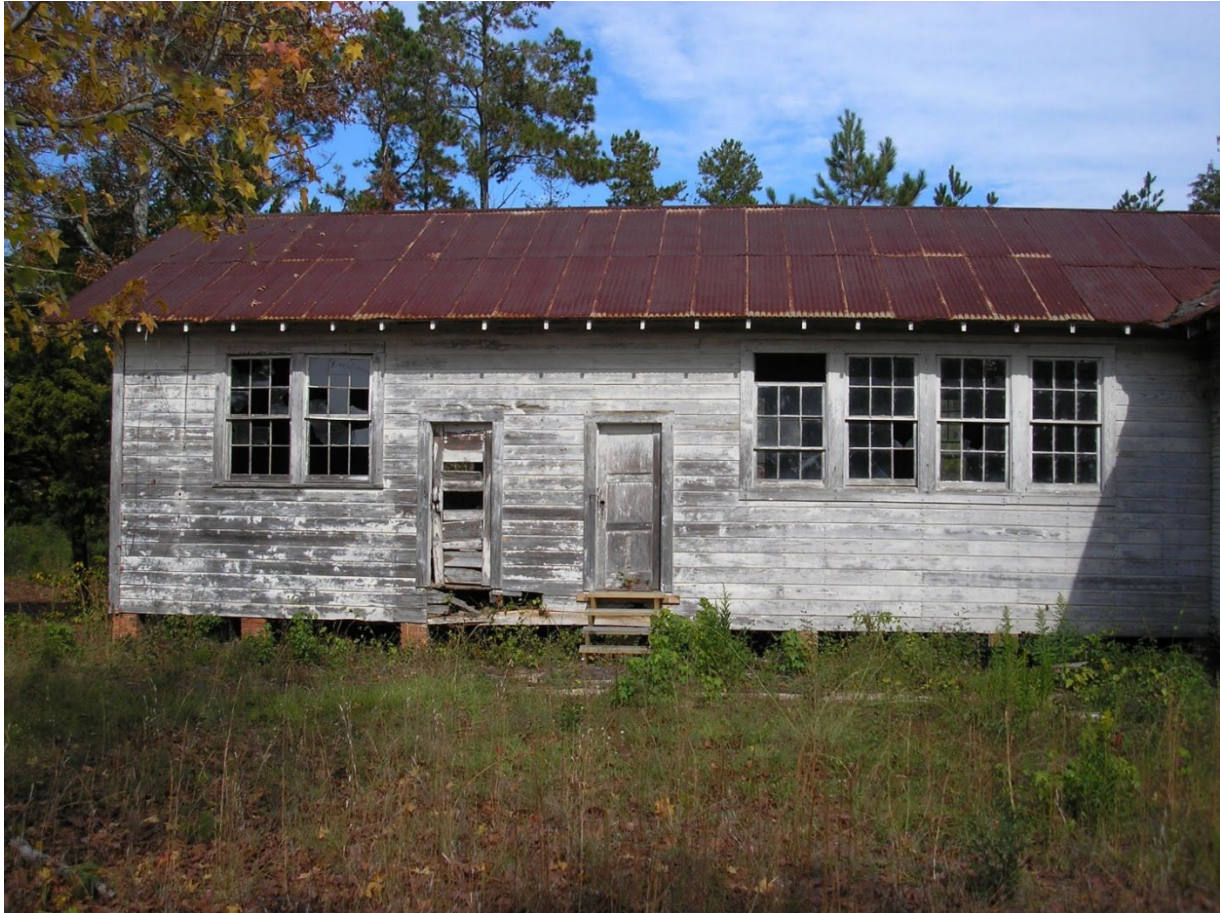
1930 West Wing, south elevation.
