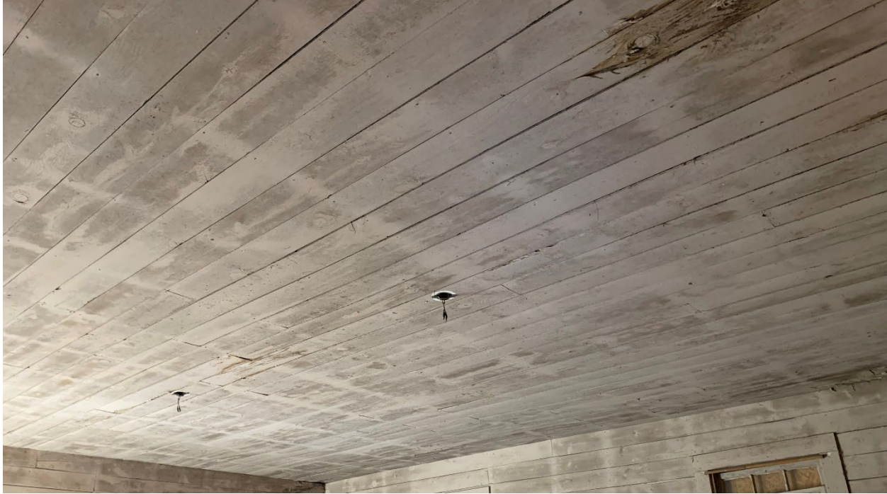
1930 West Wing. Typical ceiling material.
