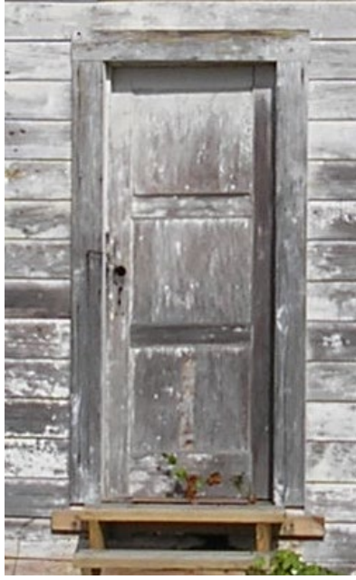
Former Door D111
