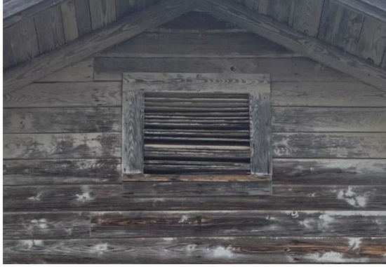
1930 West Wing. West elevation. Attic ventilation.
