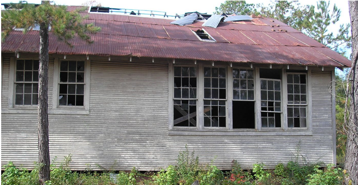
1925 Building, east elevation, north area.
