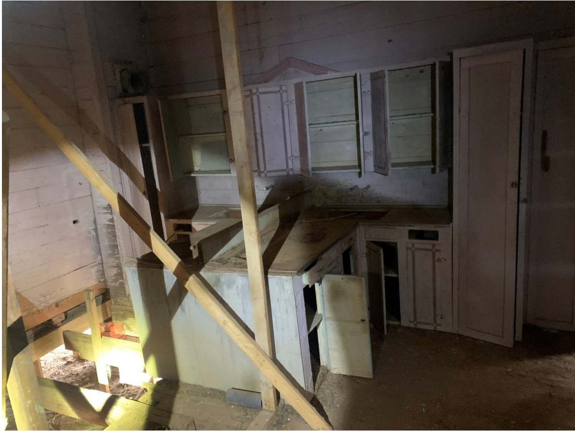
1925 Building. Room 104 – North end of room. 2023 photograph.
