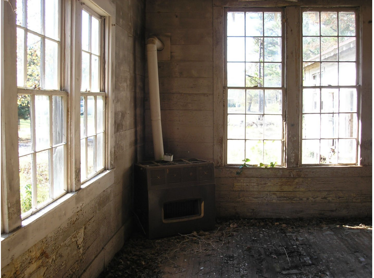
Former Space Heater (second generation heat system).
