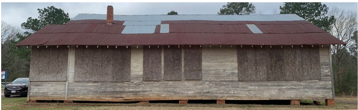
1925 Building. Roof patching and historic material.
