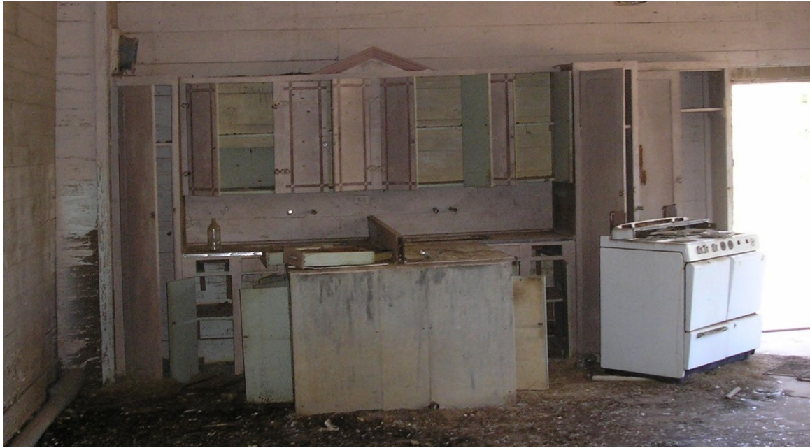
1925 Building. Room 104 – North end of room. 2008 photograph.
