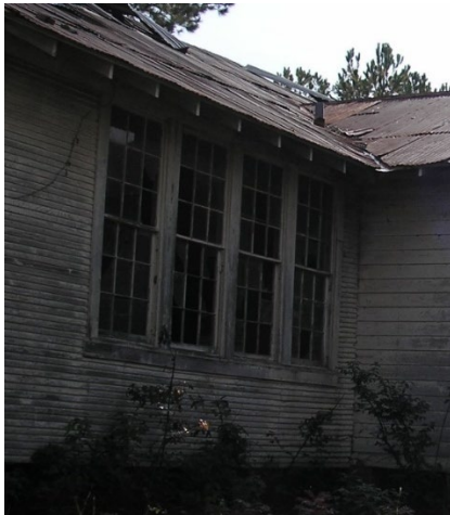
1925 Building, west elevation, north area.
