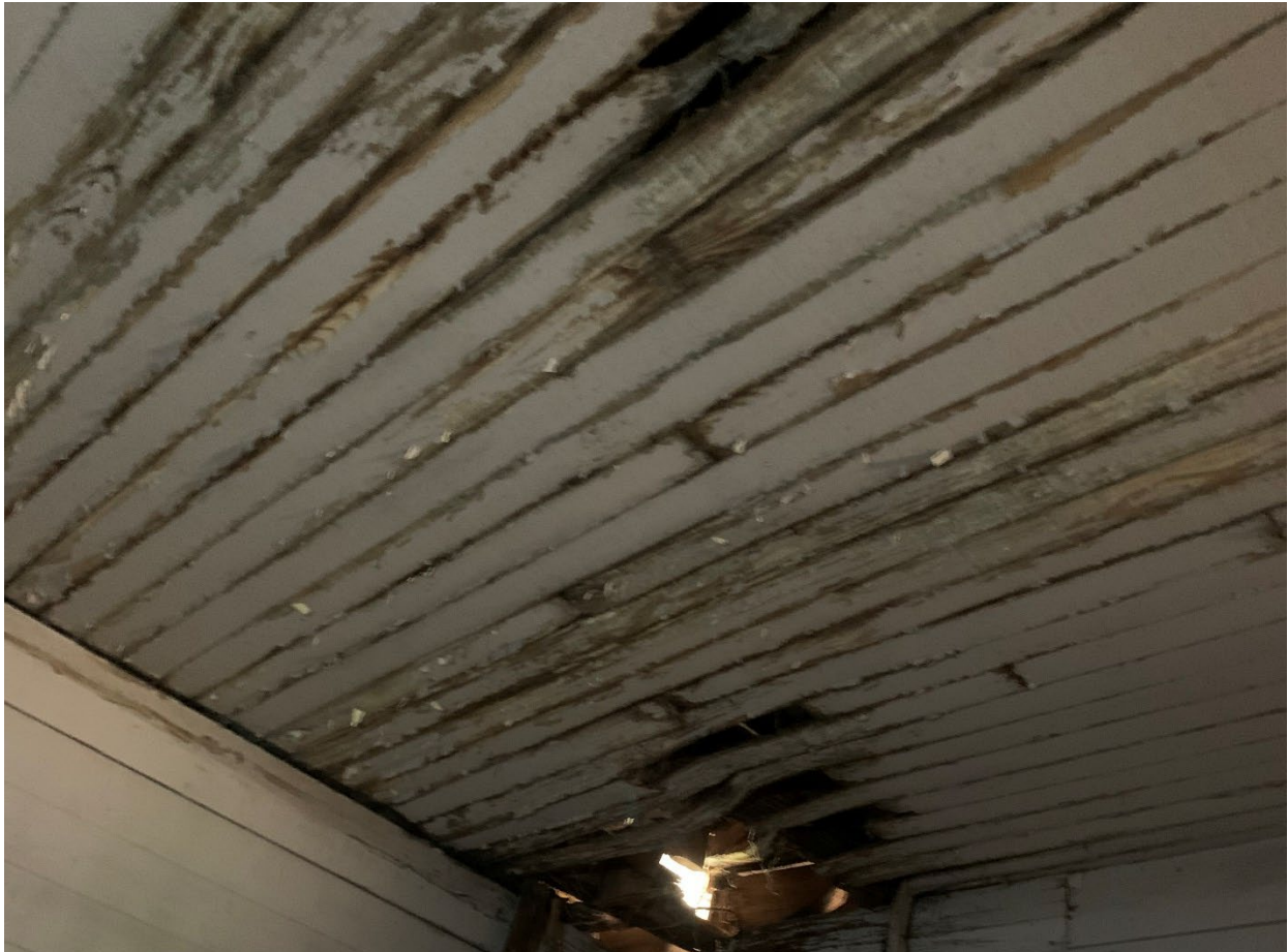
1925 Building. Typical ceiling material.
