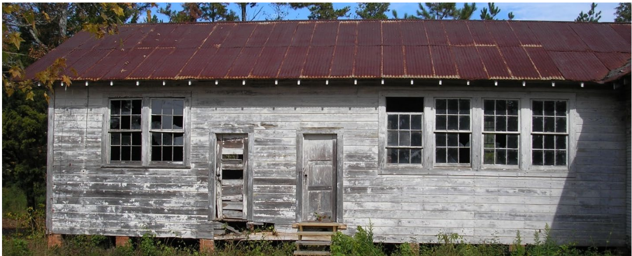
1930 West Wing. 2008 photograph.
