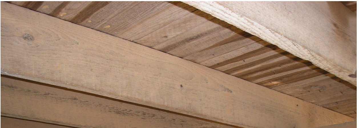
1930 West Wing. Subflooring visible from crawl space.
