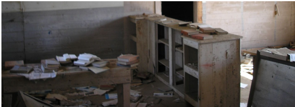
1930 West Wing, Room 111. 2008 photograph.
