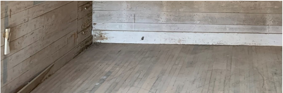
1930 West Wing. Oak flooring.
