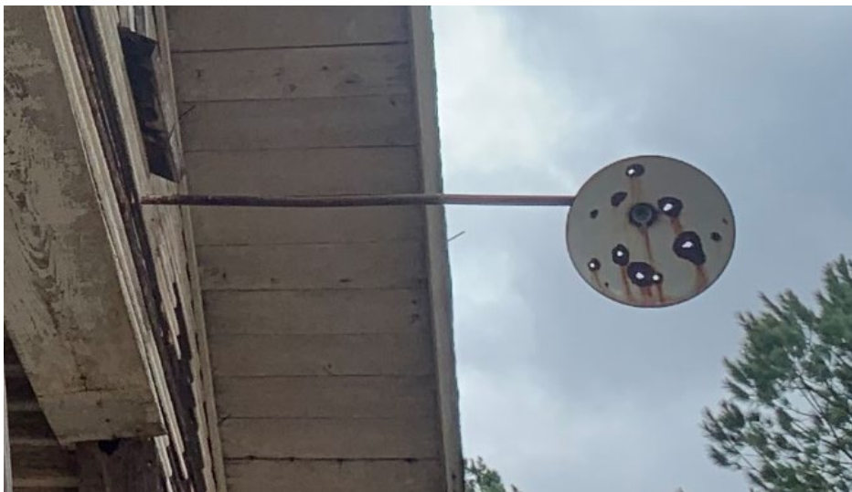
1925 Building. South elevation. Exterior light fixture.
