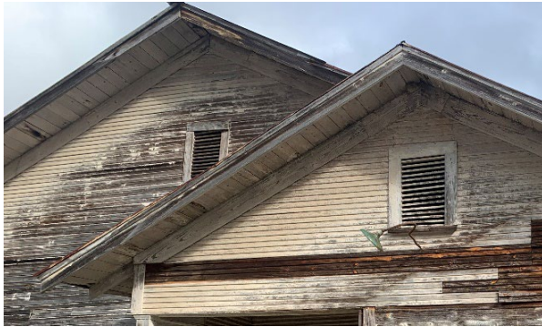
1925 Building. South elevation. Attic ventilation. 1925 Building. North elevation. Attic ventilation.
