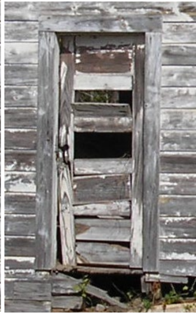
Former Door D112
