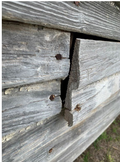
Detail of siding.
